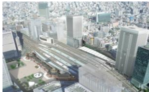
Re-development around station(1)
