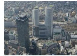
Re-development around station(2)
