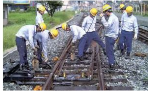
Rail track maintenance
